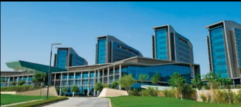
Acquisition of Sheikh Shakhboub Medical City (SSMC)
